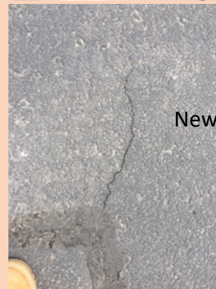
Crack in flooring in HVO
